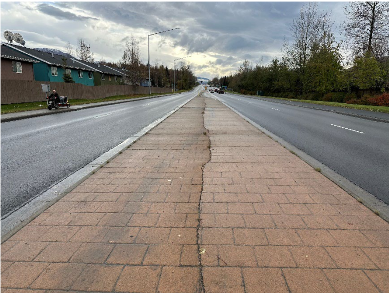
Figure 6.4 – Muldoon after sweeping operations.
